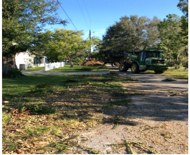
Hurricane Irma Debris Clean-up
